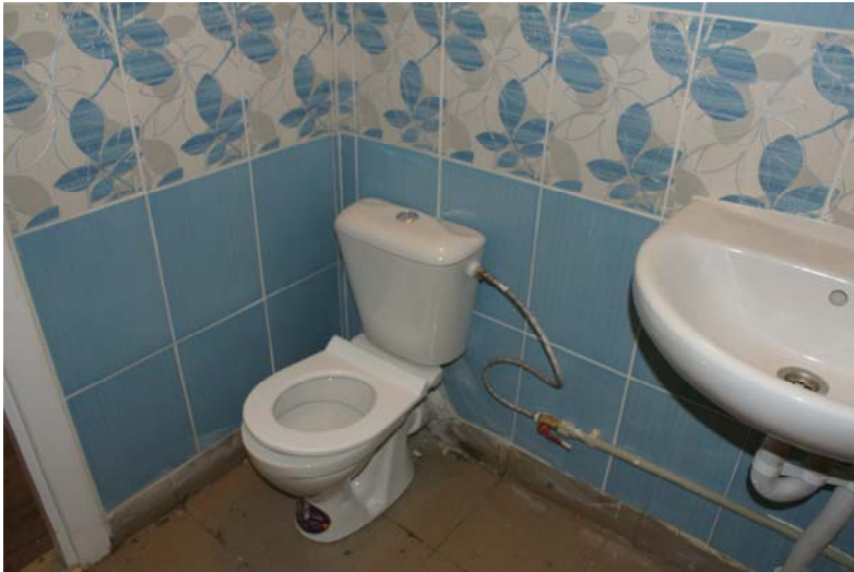
the newly tiled bathroom.....
